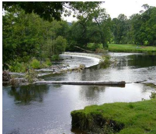
*Horseshoe Falls. The feed to the Llangollen Canal is off the bottom left corner of this image. A floating tree trunk is secured by chains across the water to prevent debris from entering the canal.*
