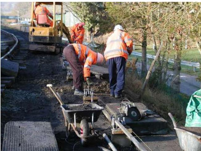
Preparing the ground for the Bomac blocks - shown to left and right of the point rods
