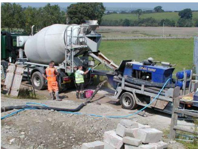
*Ready Mix and concrete pump prepare to deliver to the trench* Photo : PR
