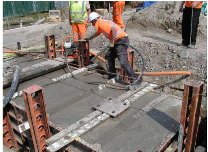
*Mike Plant adds final touches to the concrete. Note one of the bolting plates in the centre of the photo* Photo : PR
