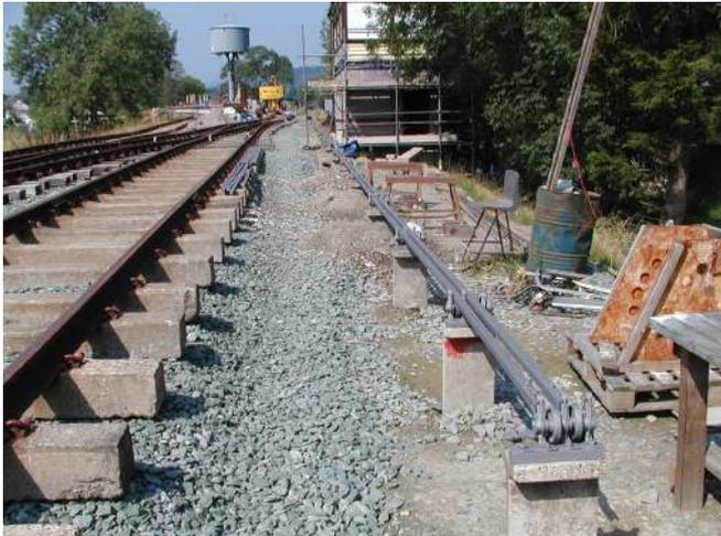
*Point rod stools and point rods in place. Notice the current gap between the rod height and ground level. This will need to be filled on each side of the stools to make for a safe walking area*
