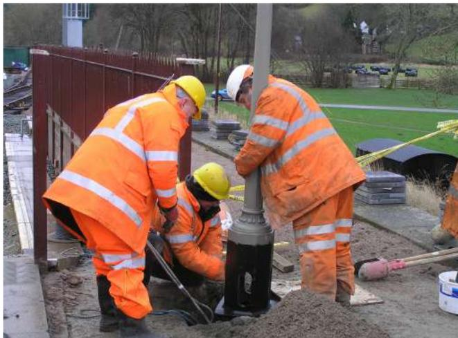
Site electrician Phil Coles cabling up a lamp post at the east end Photo : PR
