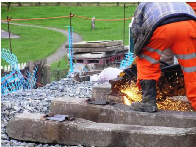
Rail saw being used to cut away old welds and to square off rail ends
