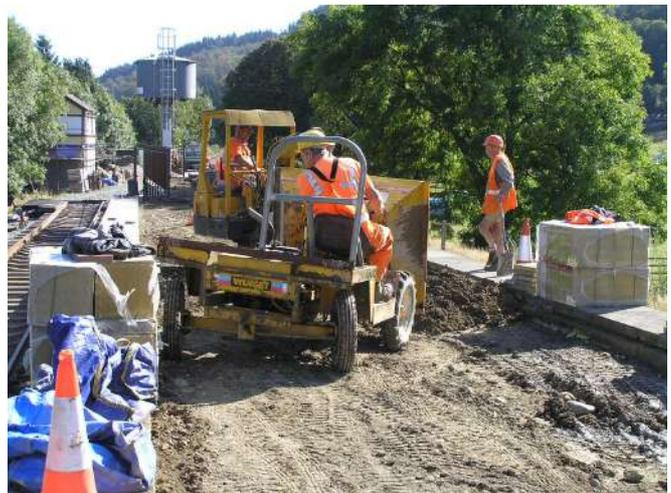
*Tipping infill at the East end. Mini digger grading-*
