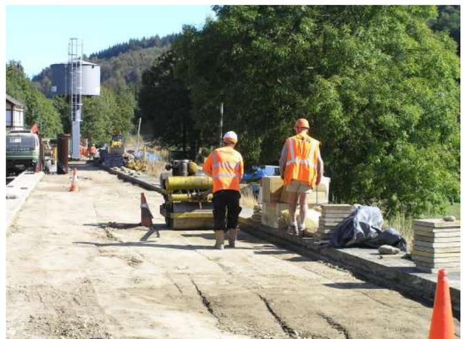
*Rolling and compacting the platform surface after the infill drop*
