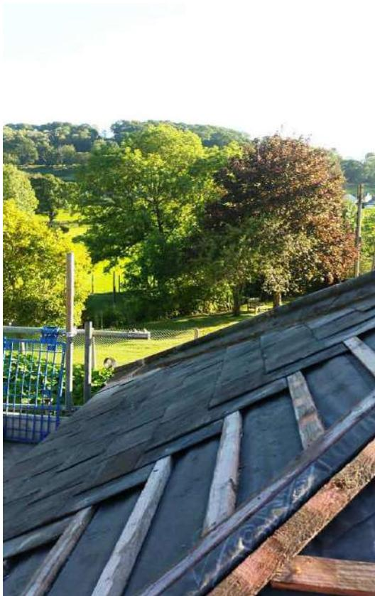
*Roof showing battens in place and slates being re-hung* Photo : PC
