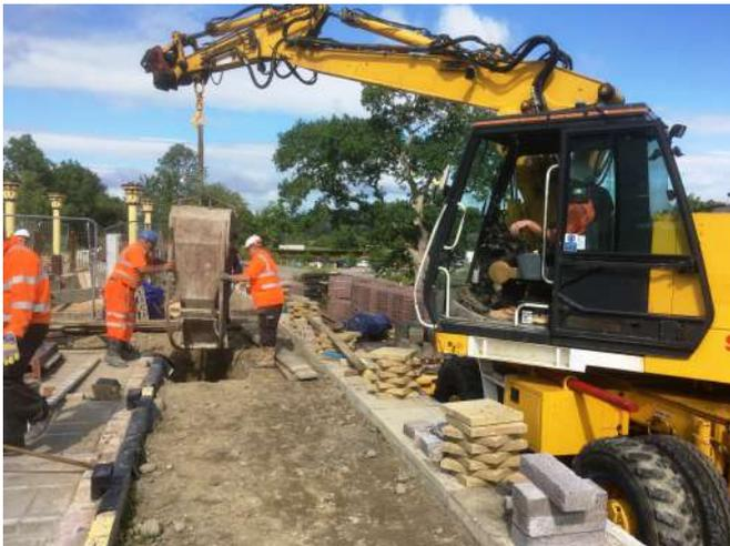
*Pouring concrete into the corner foundations using a concrete skip. The Readymix machine is behind the rail crane and can no longer get up to the site Photo : PR*
