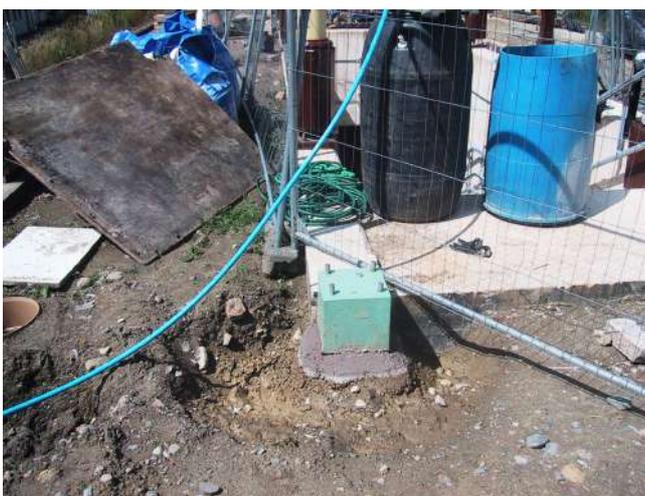
*Corner post support is now concreted into place. The new steel work will be bolted to the support shown in green Photo: PR*
