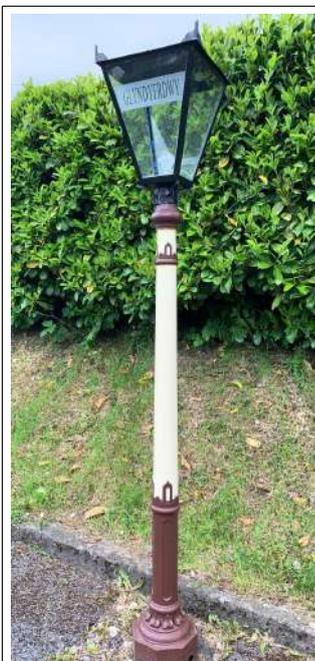
The above photo of Lamp post shows the correct pattern for the casting. The lantern top, although rather "smart" is not the "correct" pattern. The authentic lantern top is shown in photograph 2 standing next to Carrog Signal Box
