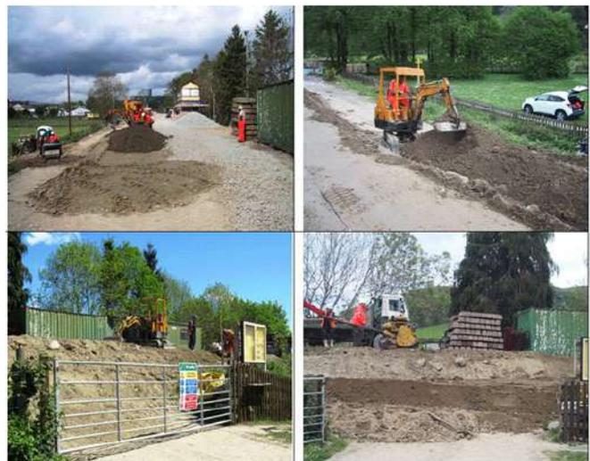
Clockwise from top left - Grading in top surface, Filling south batter, Layering and rolling, - almost complete, Gap filled - new 3 metre batter bars the way Photos : GJ and PR
