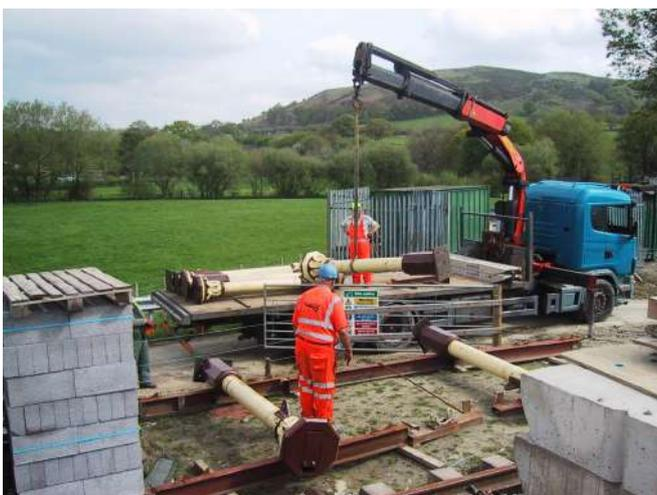
*Columns being unloaded showing counter balances and base plates* Photo : PR
