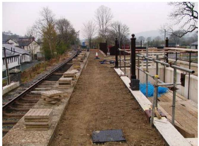
*West end single platform levelled and ready for tamping down* Photo : PR
