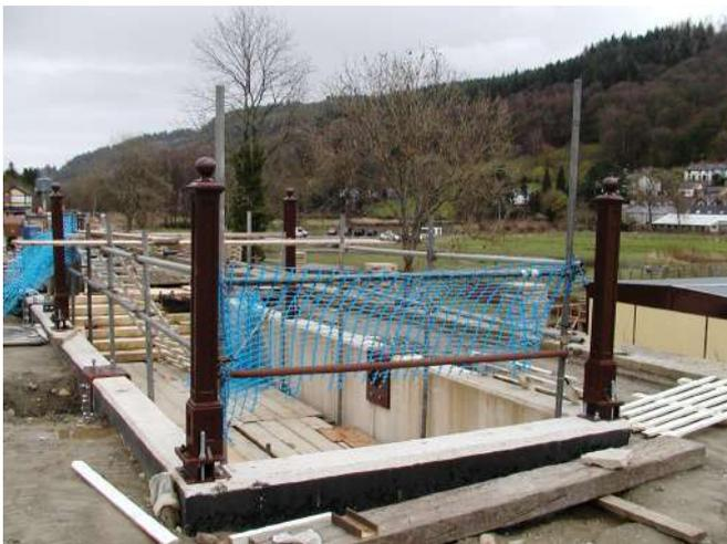
*Corner posts in place at the top of underpass. Column saddles in between the posts Photo : PR*
