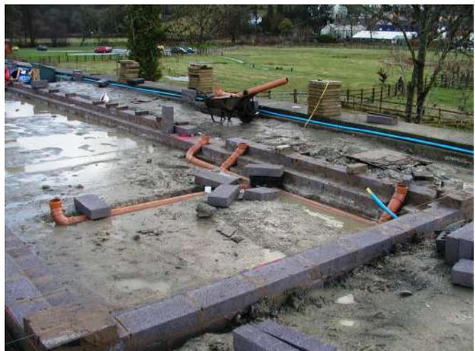
Sewer pipes being installed in the platform waiting room
