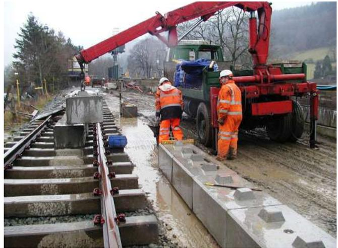
*Easi Blocs being added to the UP platform wall Photo : PR*
