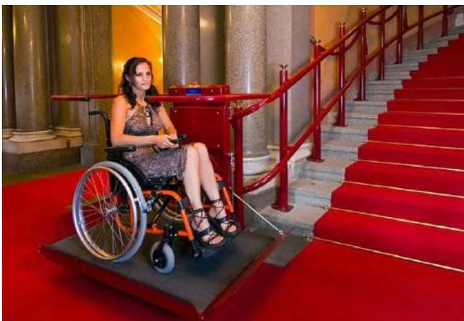
*Wheelchair platform lift of the type to be fitted to the underpass stairs with passenger ready to ascend*
