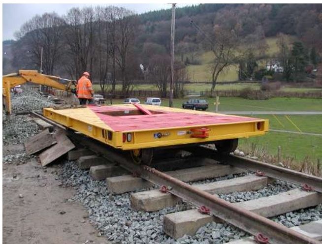
P-way trailer on site at Corwen Central Photo : PR
