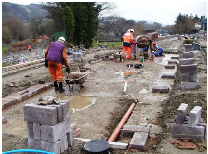
First blocks for platform building Photo: PR
