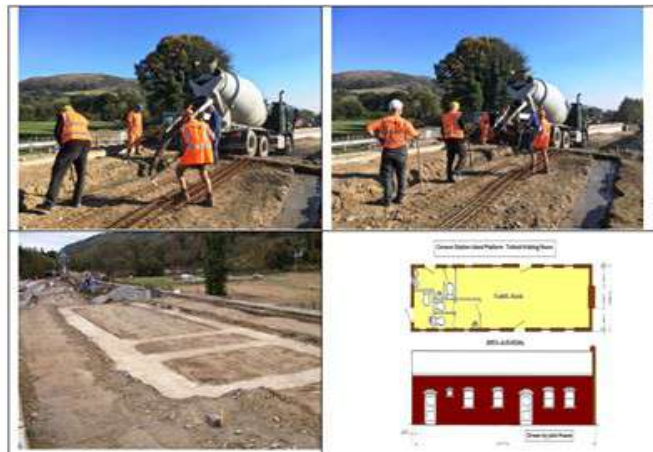
(L-R) Running concrete into footings ground plan, completed footings Photos : GJ/PR
