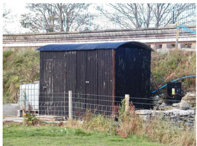
Pump House complete with newly painted roof
