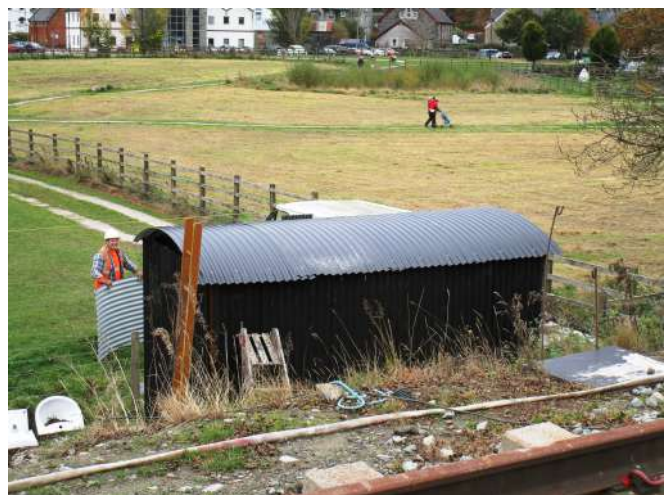
Peter Neve inspects the Pump House roof
