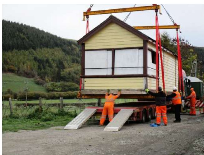
Signal Box lowering on trailer at Carrog Yard Photo : GJ
