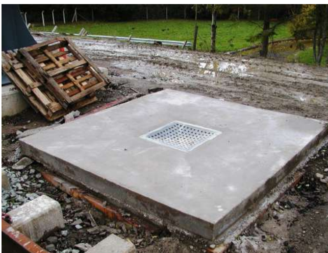
Water Tower overflow drain
