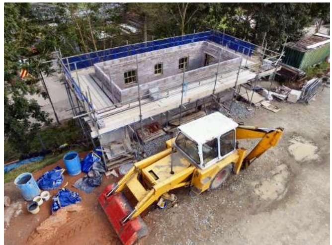
Drone view of completed locking room
