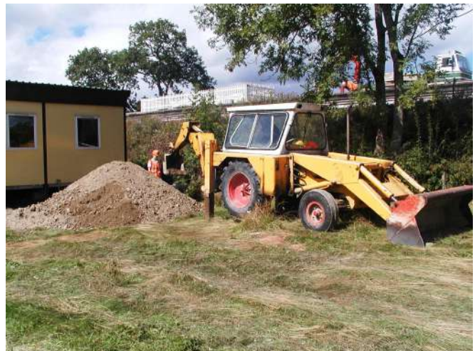
Ground works for station building access Photo : PR
