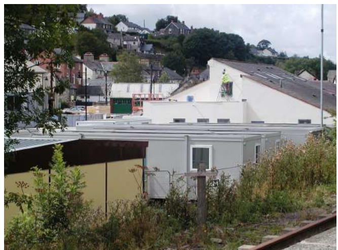
New Health Centre rises above temporary "Health village" Photo : PR
