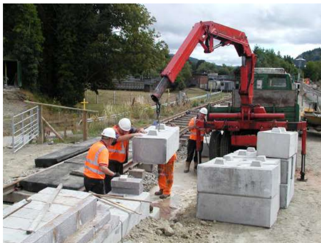
Easi-blocs approaching Ruthin Spur crossing Photo: PR
