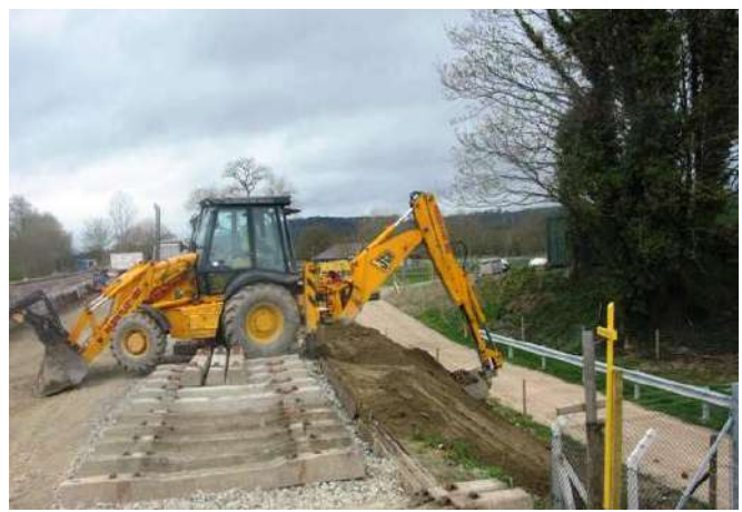
Grading in and extending the North Batter Photo: PM
