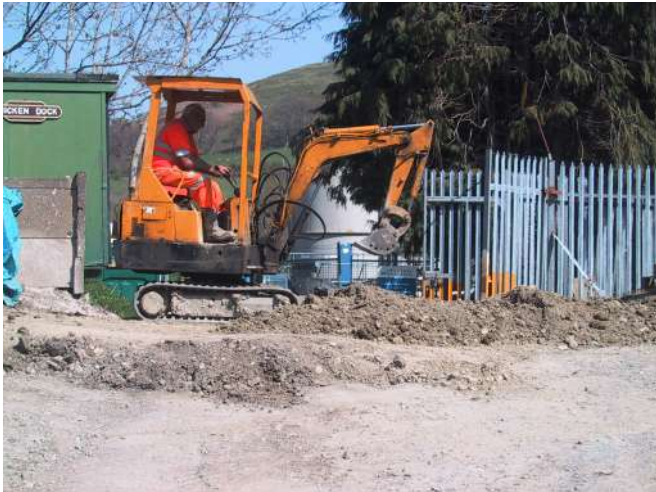
Reducing the dip. Mini digger grading in Photo: PR
